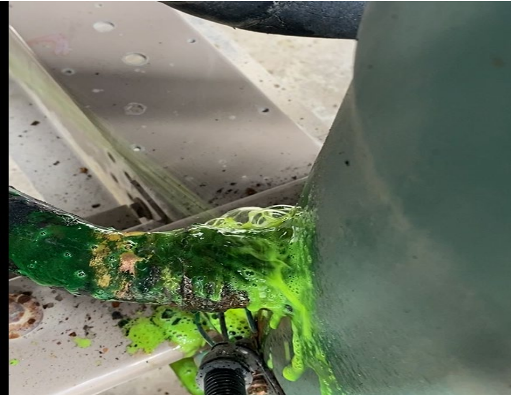
COMPRESSOR FREON LEAK
