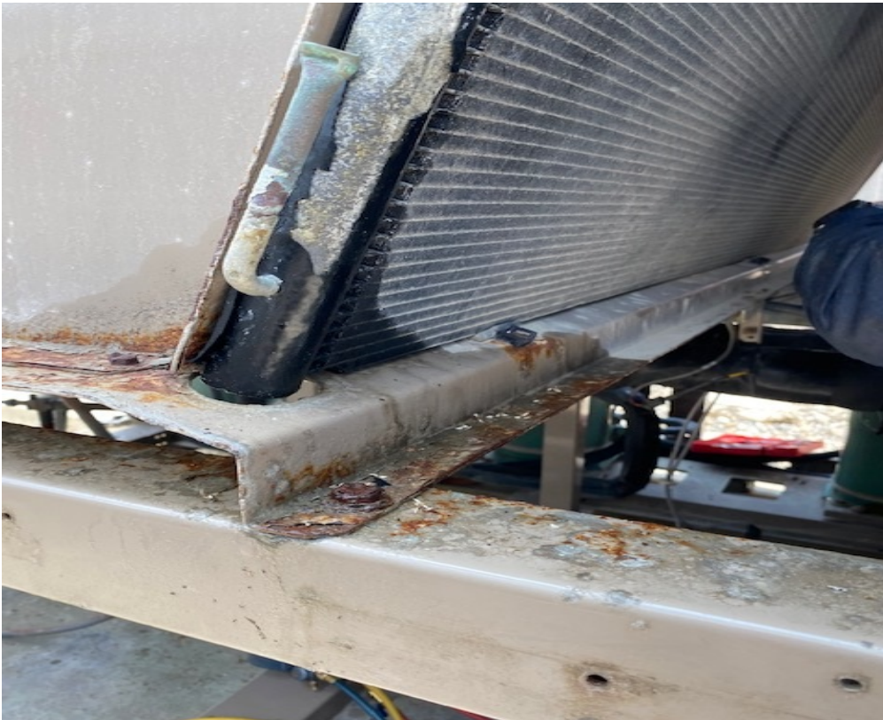
COIL FREON LEAK
