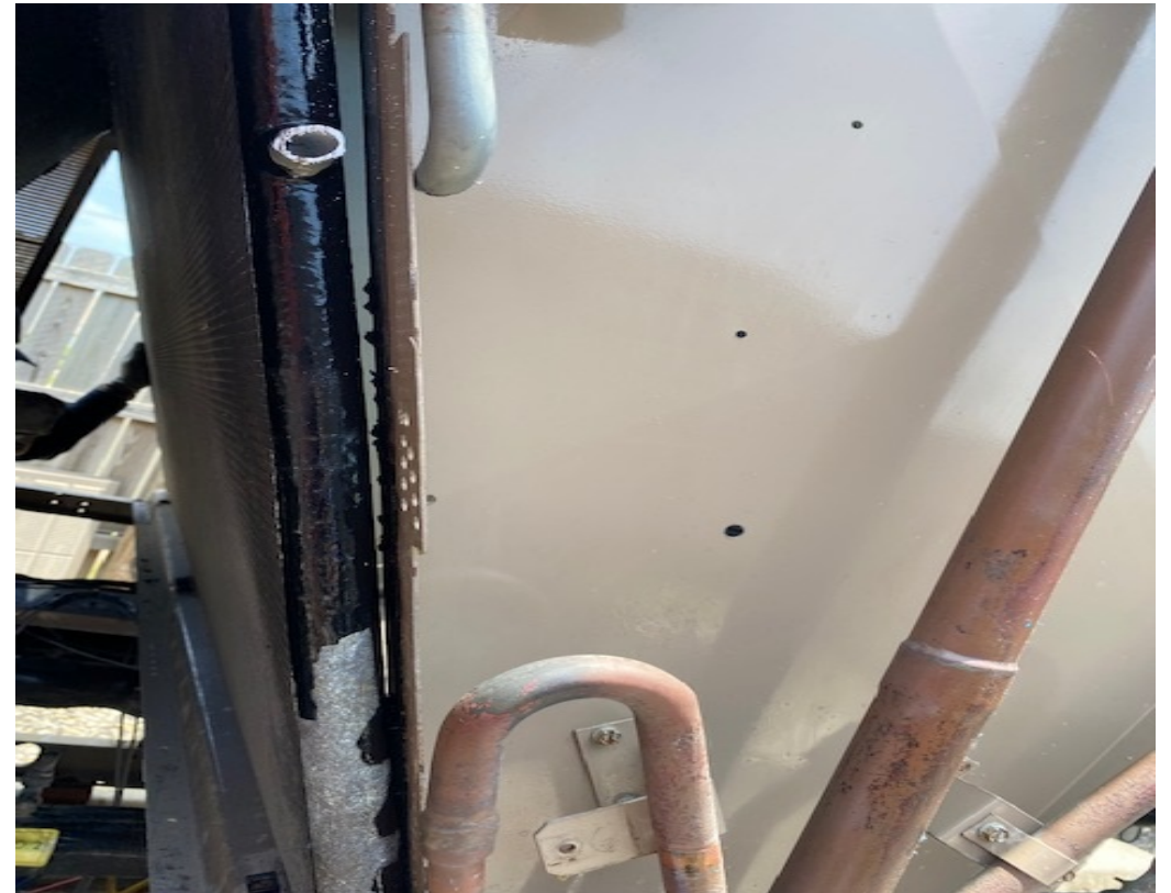
COIL FREON LEAK
