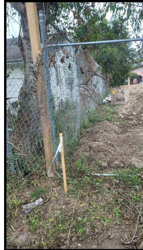
Figure 8. Wood Pole Field Staking
