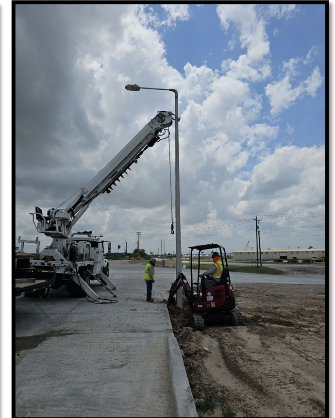
Figure 9. Street Light on Concrete Pole Install
