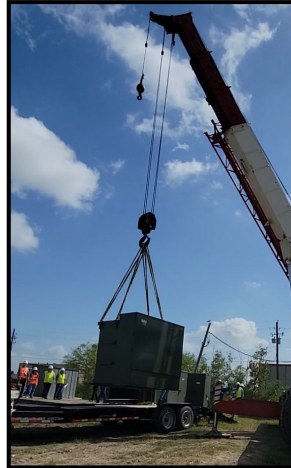
Figure 5. Transformer Install
