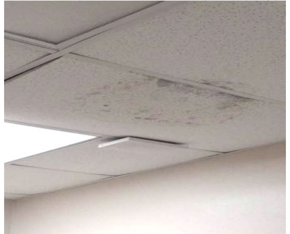
MOLD GROWTH ON CEILING PANELS
