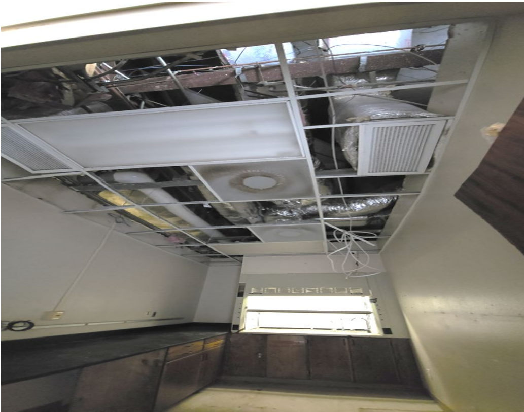
REMOVAL OF CEILING PANELS
