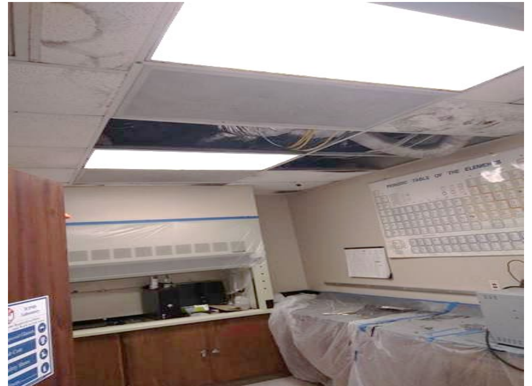
MOLD GROWTH ON CEILING PANELS
