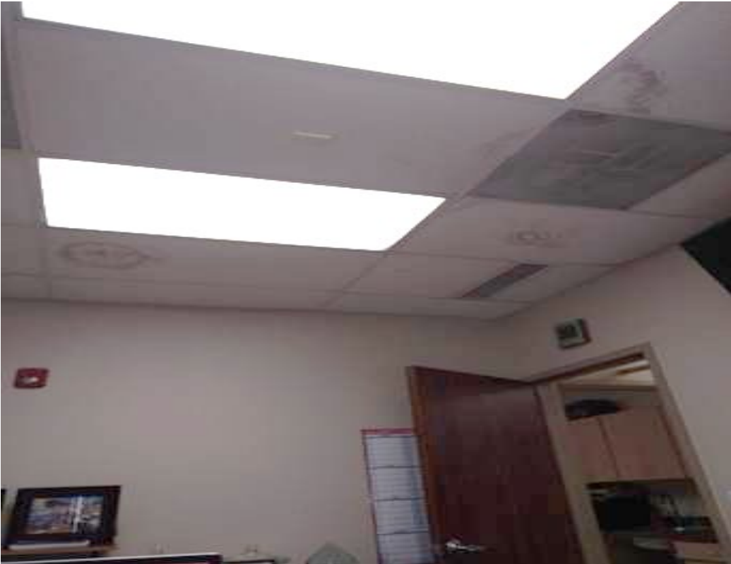
MOLD GROWTH ON CEILING PANELS
