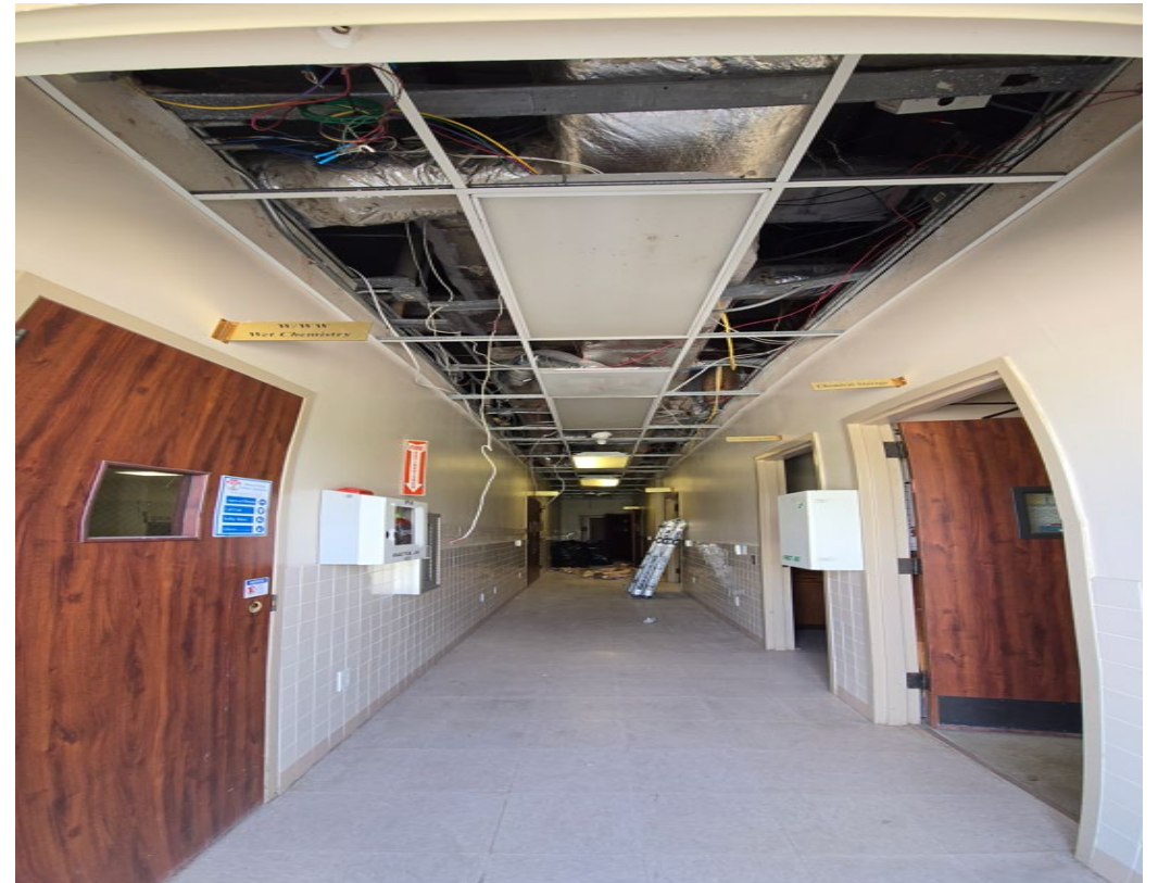
REMOVAL OF CEILING PANELS
