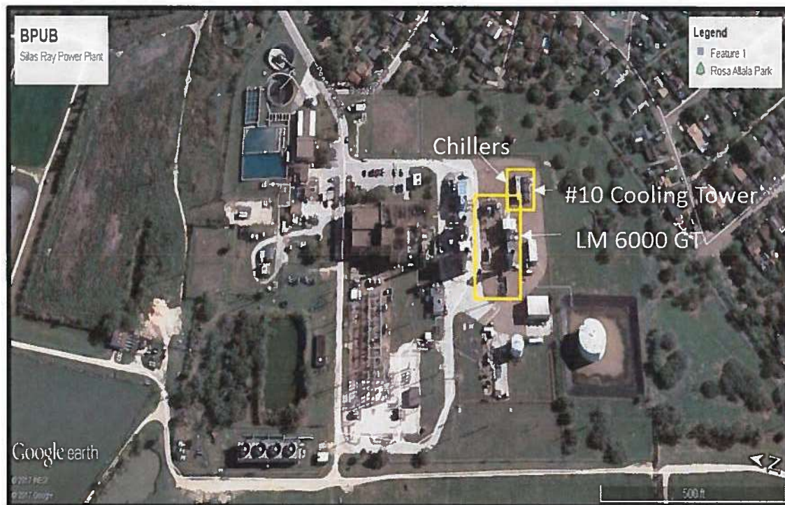
Figure 1 Silas Ray Power Plant LM6000, Chillers and #10 Cooling Tower Arrangement
