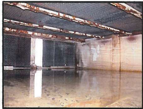
Picture 2 Typical condition of internal cross members supporting the fill system. The Facility reports that these cross members have been replaced previously.
