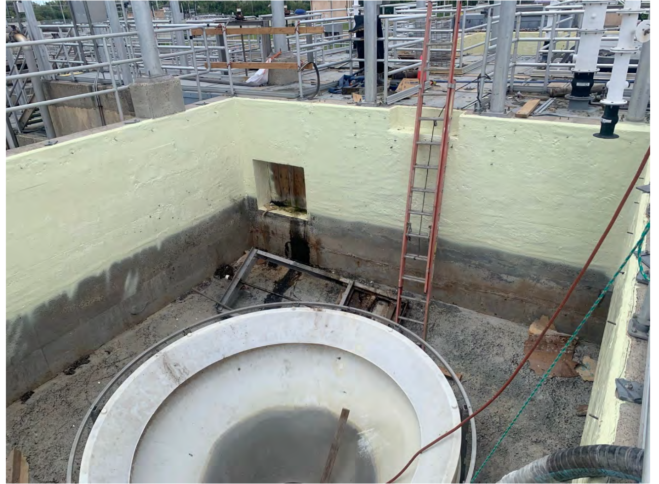
New Grit Basin Coating and Headcell Installed
