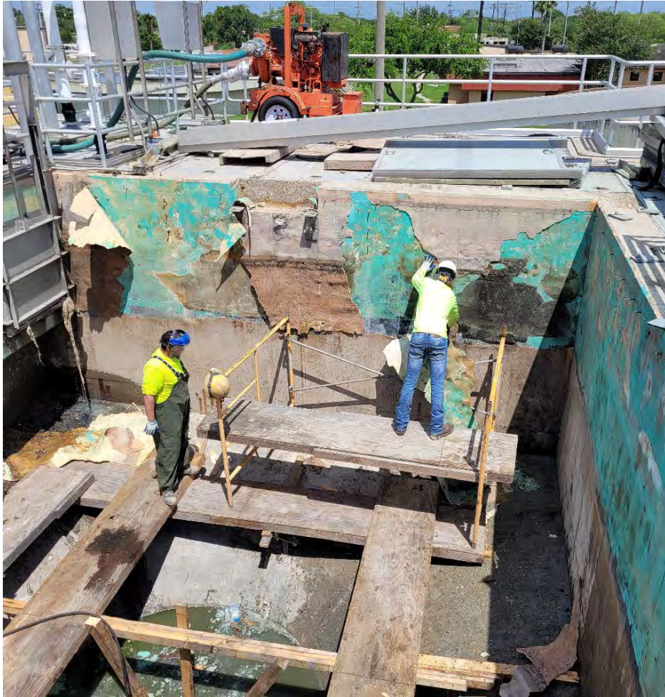
Grit Basin Coating Removal
