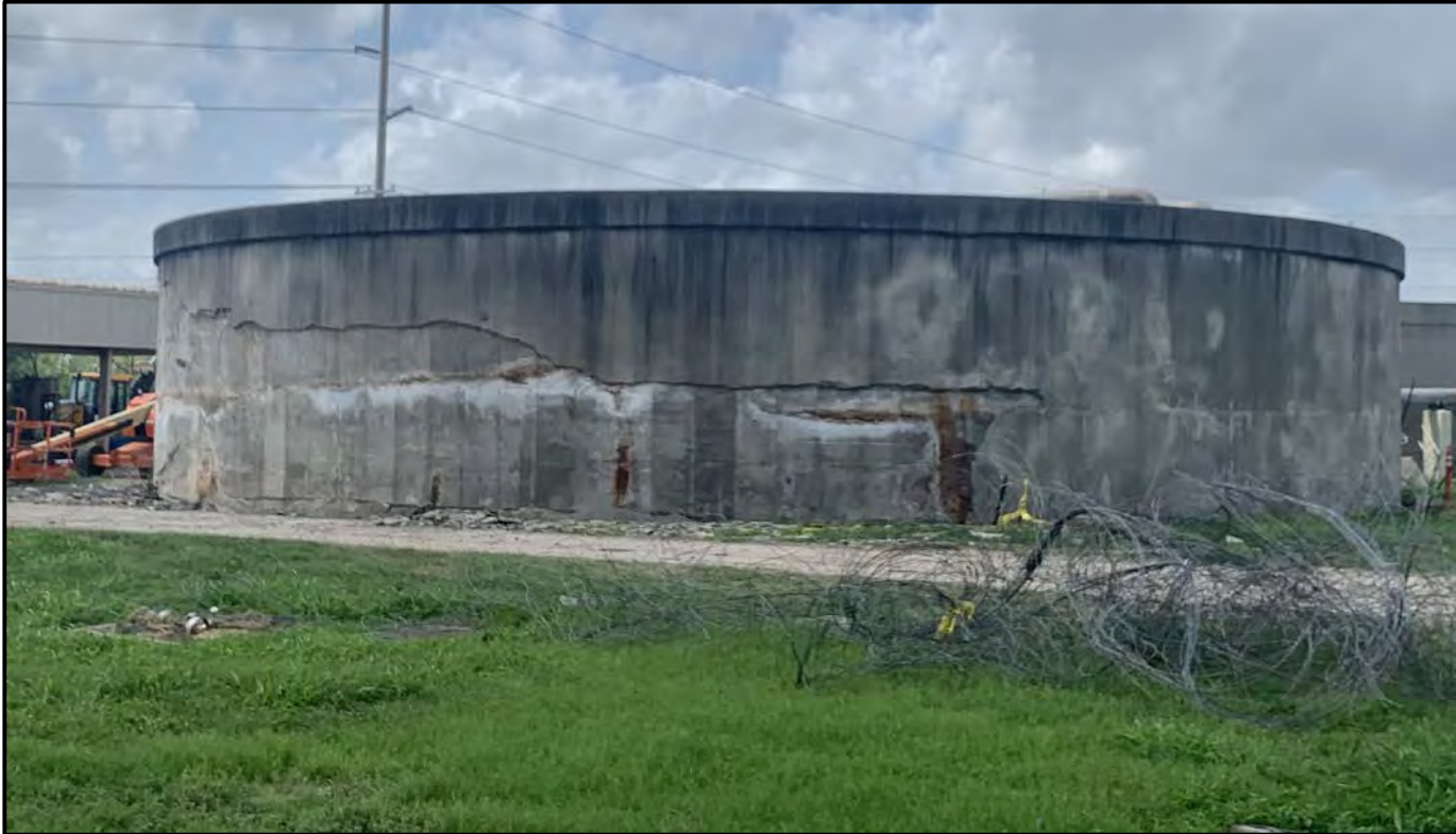
Digester No. 1 Shotcrete and reinforcement removal
