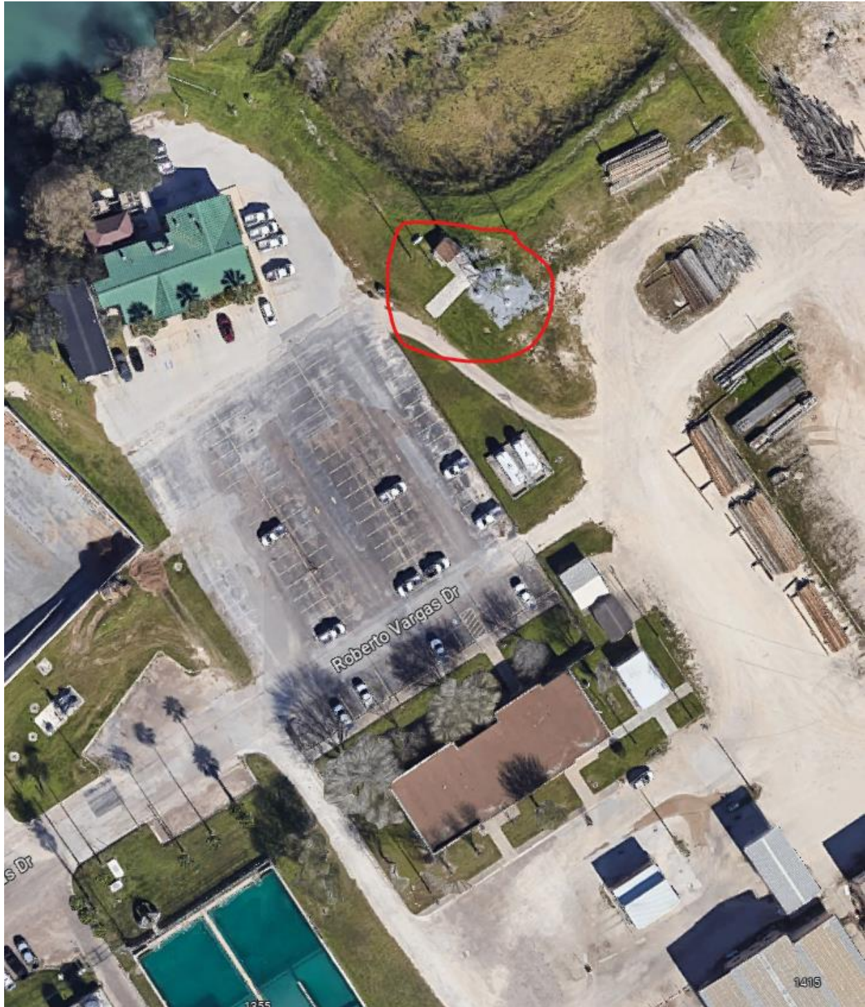
Figure 2: Tower & Shelter Location in BPUB Compound
