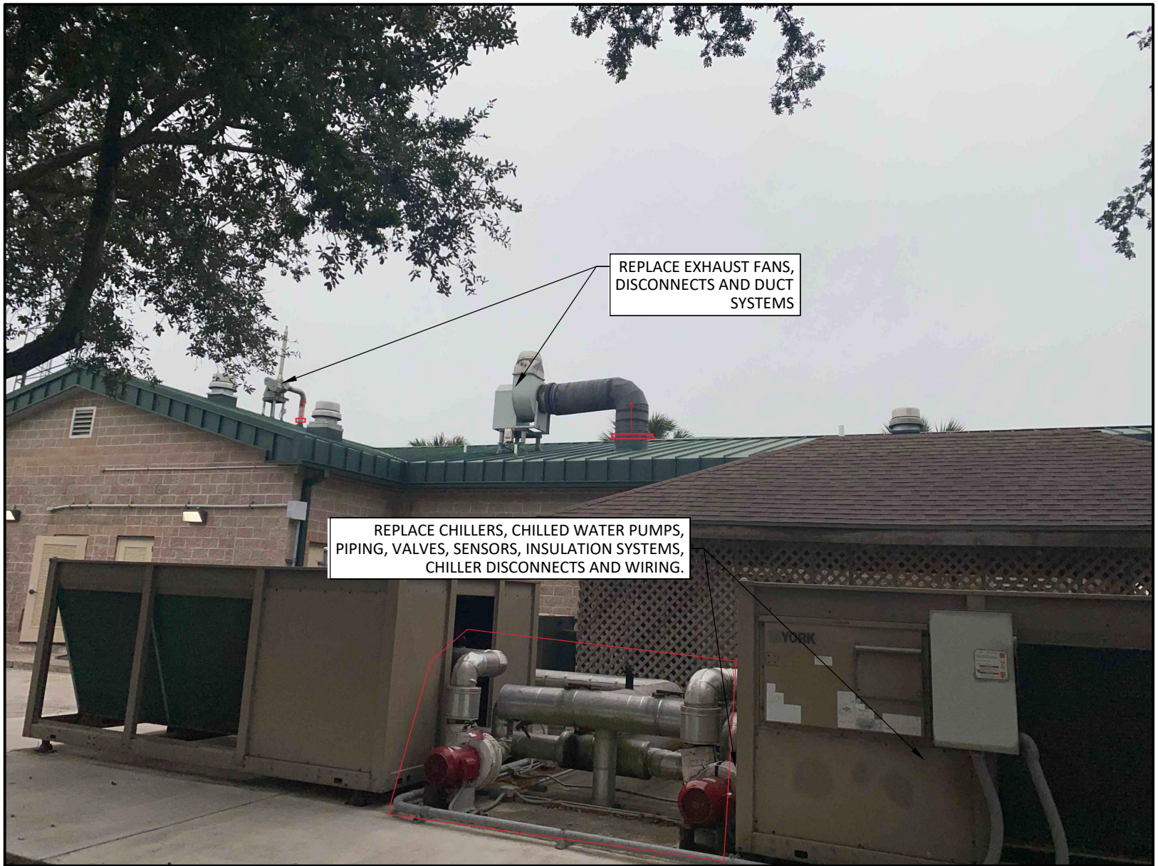
47 16 EXTERIOR CHILLERS AND ROOFTOP EXHAUST FANS
