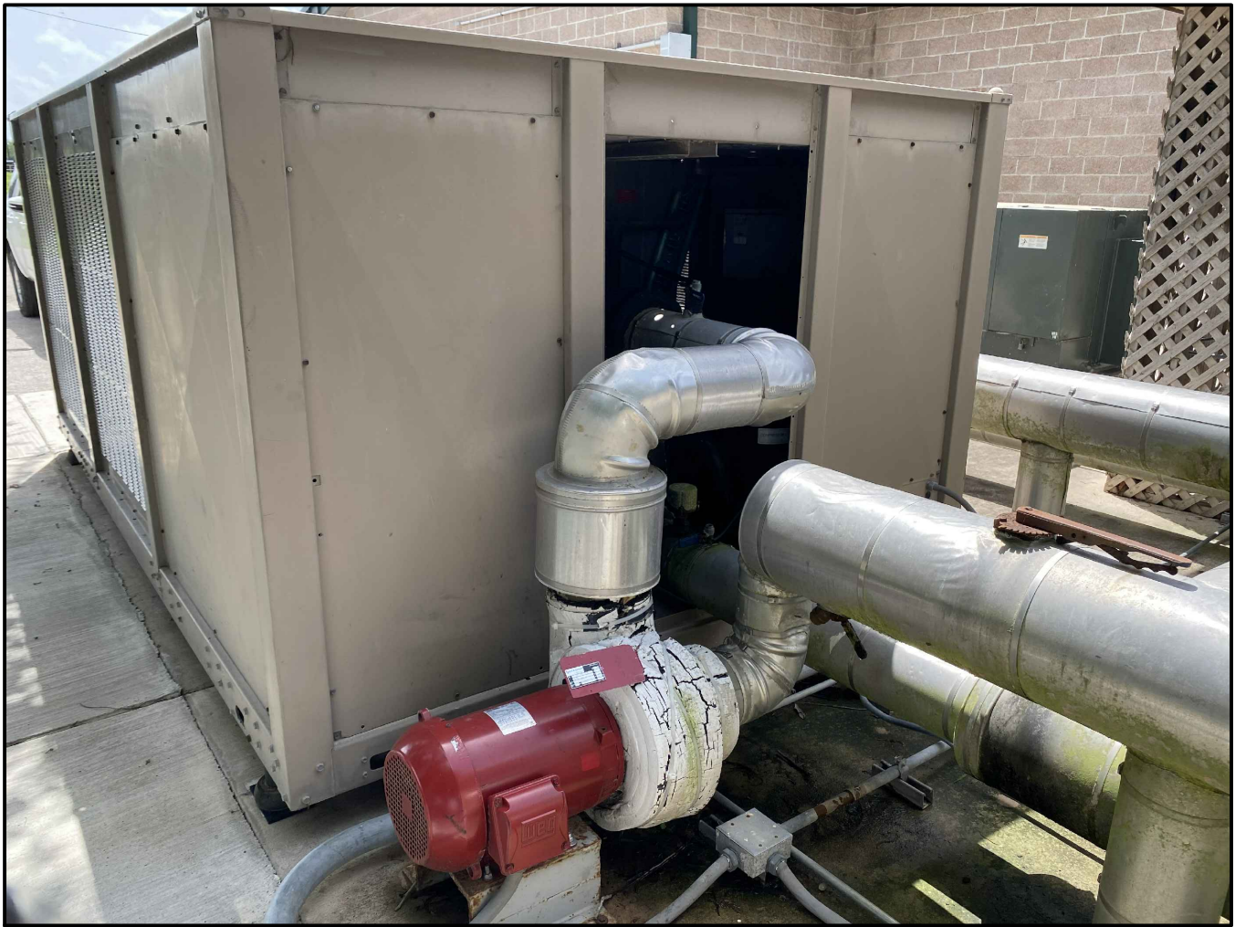
38 15 ACC-1 AND CHILLER PUMP P-1
