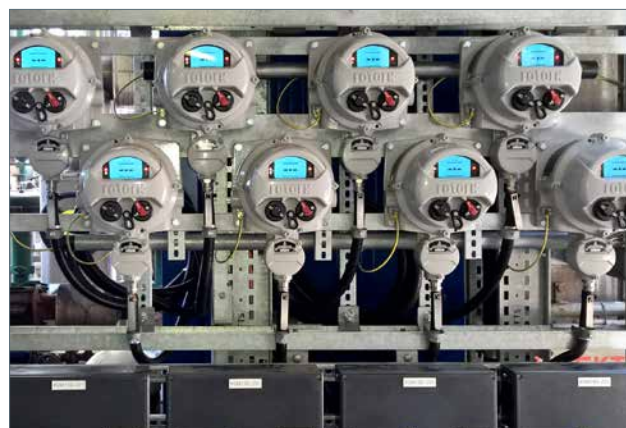
RHS operating IQ and SI actuators in inaccessible locations
